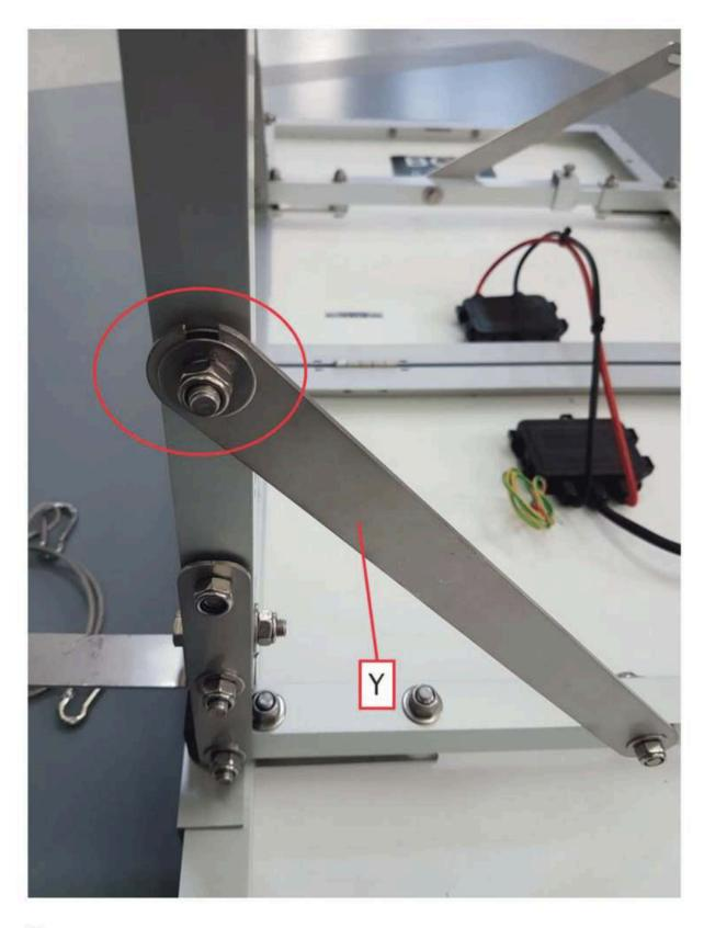
7. Put the diagonal bracket (Pos. Y) in between the 2 rings, and screw the nut tight.
