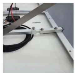
4. Put the brackets on the edges of the panels, and extend them so they fit (marked red).
