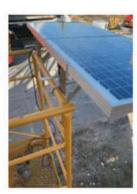
8. Place the solar panel on the outside of the basket. Let it rest on the 2 U-formed strips (Pos Z).
